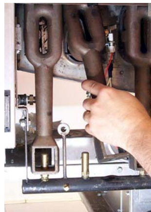
Removing burners from rethermalizer.
