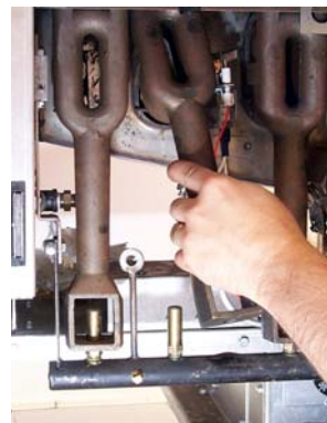
Remove burners to gain access to temperature probe.
