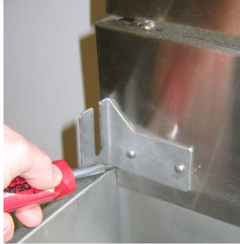
Removing flue cap.
