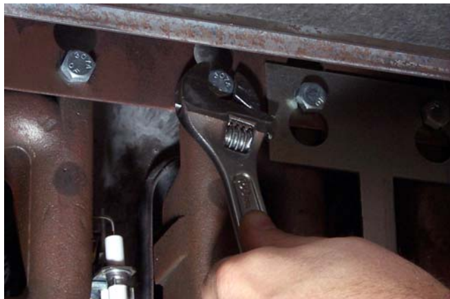
Loosening burner bolts prior to burner removal.
