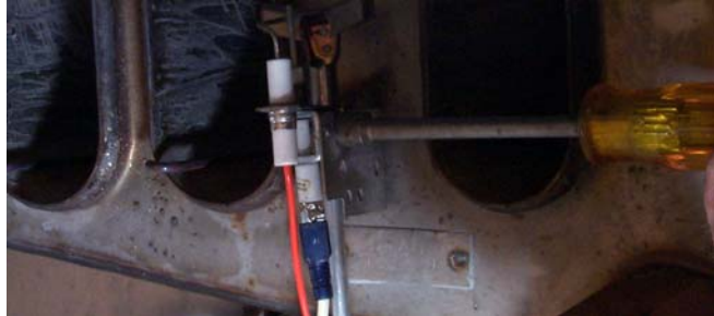
Removing electronic/standing pilot assembly.
