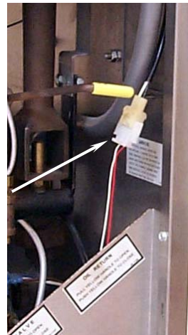
Disconnect the two-pin probe harness connector (arrow).
