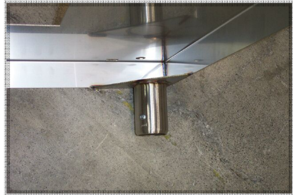
Figure 1—Leg socket showing set screw
