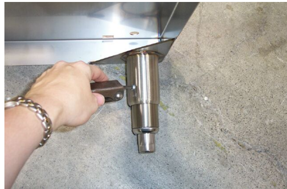
Figure 2—Tightening the legs
