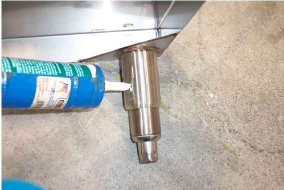
Figure 3—Applying silicon
