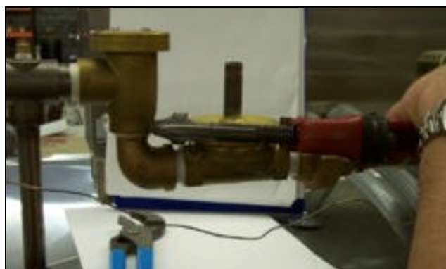
Loosening the valve bonnet
