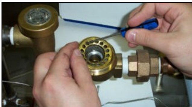
Removing the screen retainer
