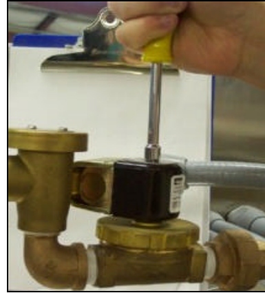
Removing the top screw
